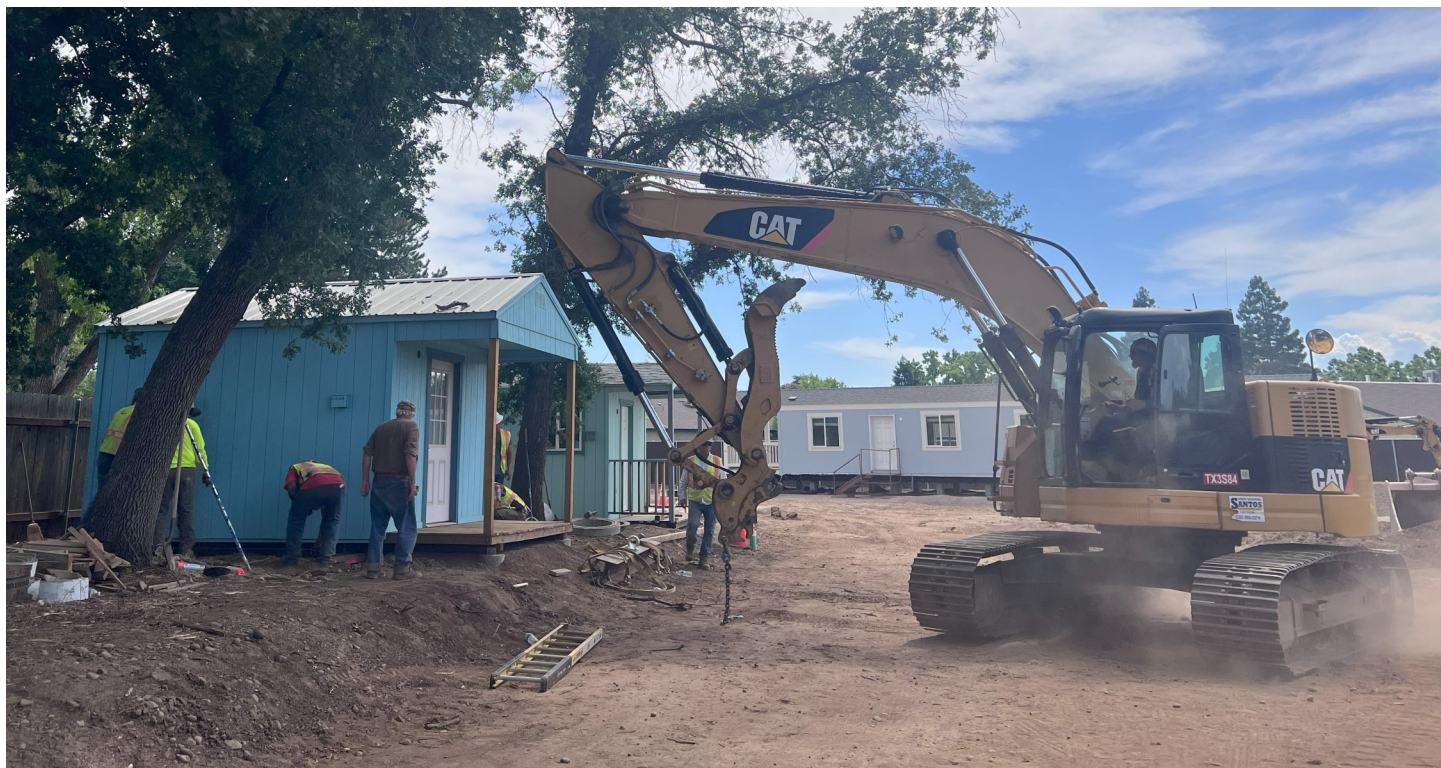
Workers place two of the 20 sleeping cabins at the Everhart Village site. The 72-foot modular community building is in the background.
